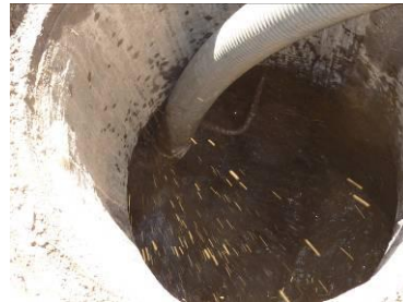
Figure 38: Discharge of collected sludge in a sewer manhole
