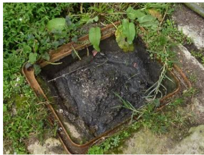
Figure 26: Accumulation of toilet waste due to blocked sewer pipes
