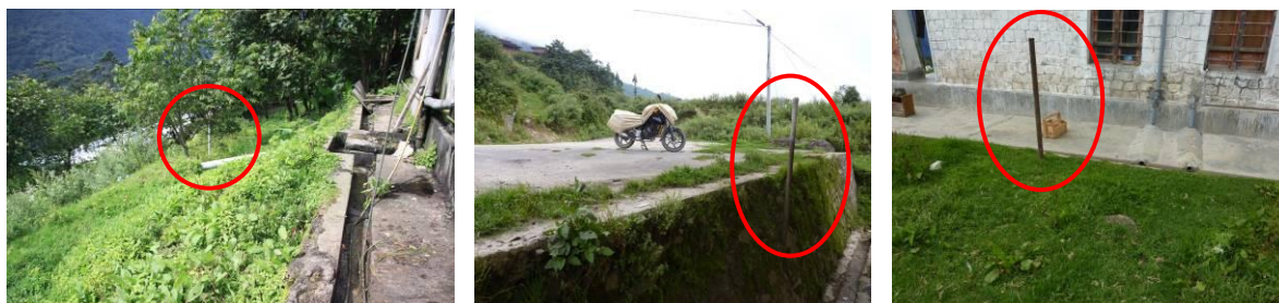
Figure 3: Difficult access to septic tanks
