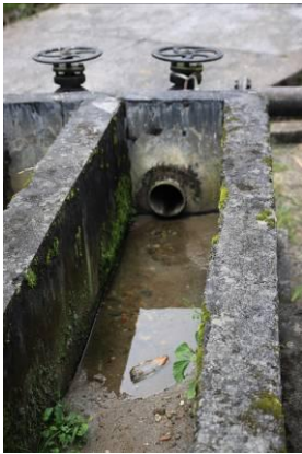
Figure 24: Inlet of the sewage treatment plant
