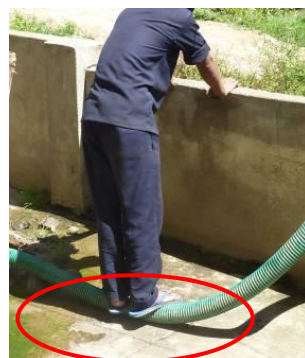
Figure 37: Improper equipment (shoes) during desludging operation
