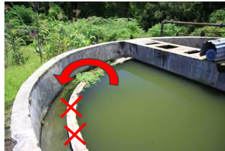
Figure 31: Irregular flow removal at the periphery of the sedimentation tank
