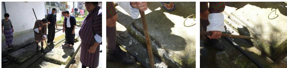
Figure 5: Opening of a sealed septic tank
