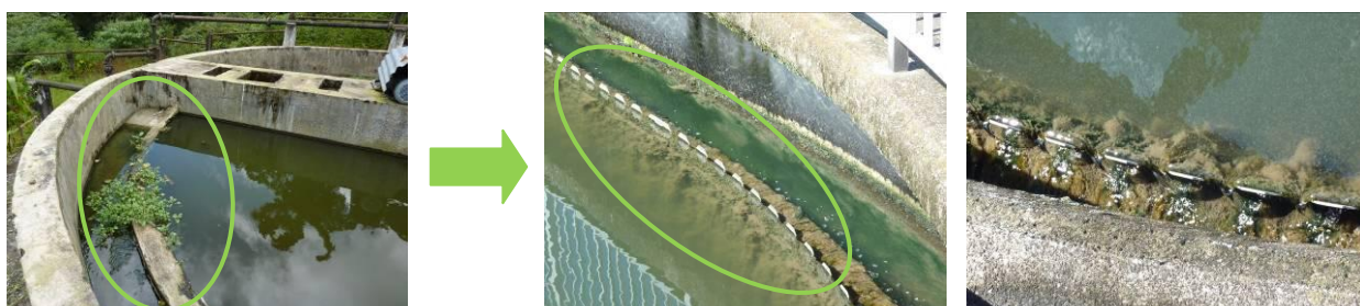
Figure 43: Appropriate outlet zone for uniform flow removal in the sedimentation tank
