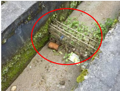
Figure 30: Actual screening system at the sewage treatment plant
