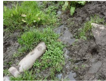
Figure 16: Broken connection between a BPC building to a septic tank downstream
