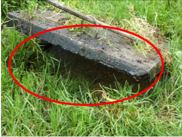
Figure 14: Overload of sludge in septic tank
