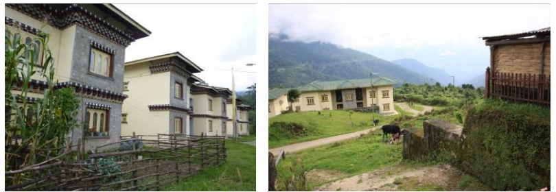
Figure 25: Student accommodations in Gedu (connected to the sewage treatment plant)
