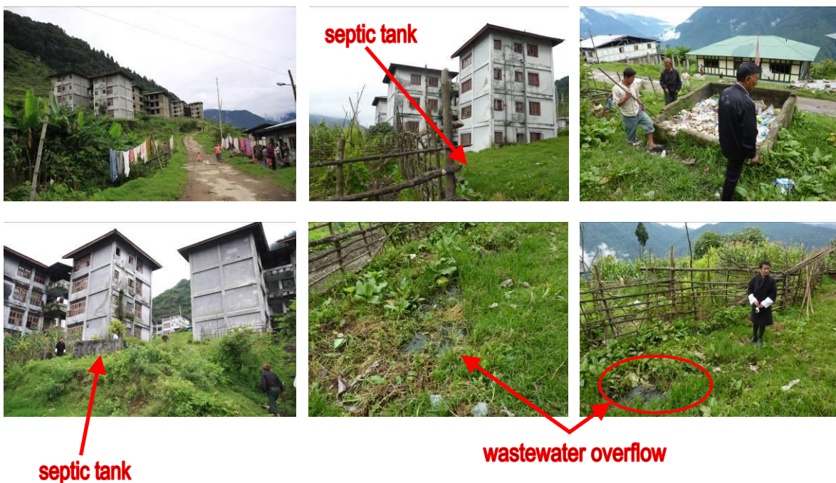
Figure 12: Unsanitary conditions at the BPC colony (Tsimalakha)
