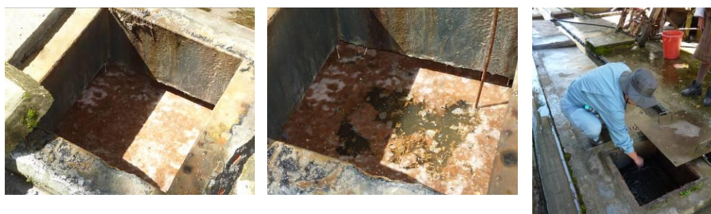
Figure 6: Absence of sludge observed in one septic tank
