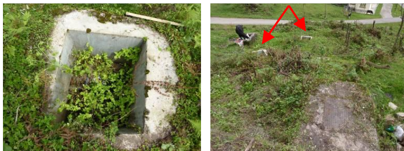
Figure 28: Sewer inspection chambers blocked due to the absence of maintenance
