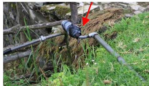
Figure 18: Repair of leak in water supply pipe
