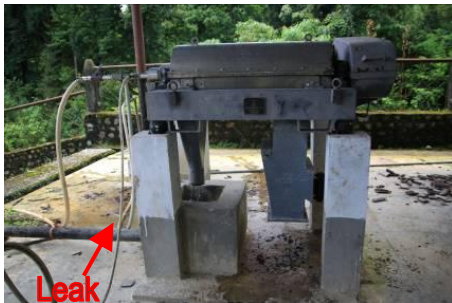
Figure 32: Maintenance issue with the dewatering machine
