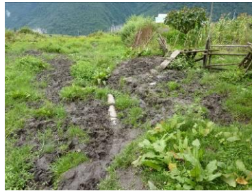
Figure 16: Broken connection between a BPC building to a septic tank downstream
