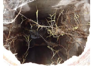
Figure 15: Empty septic tank
