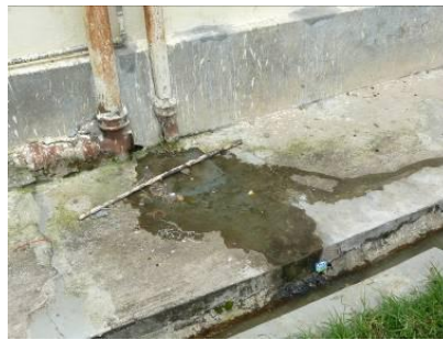
Figure 27: Grey water overflowing from inlet
