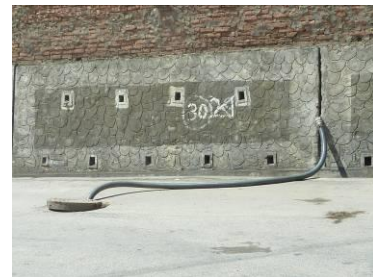
Figure 39: Potential danger with traffic after discharge operations
