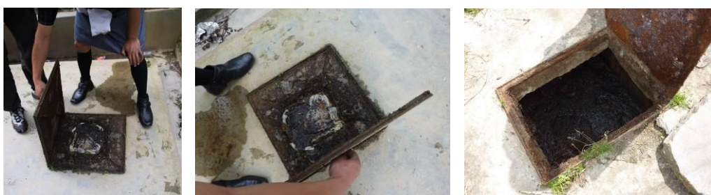
Figure 4: Accumulated sludge in septic tanks
