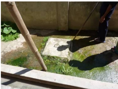
Figure 35: Septic tank before desludging operation in Thimphu (visible wastewater overflow)
