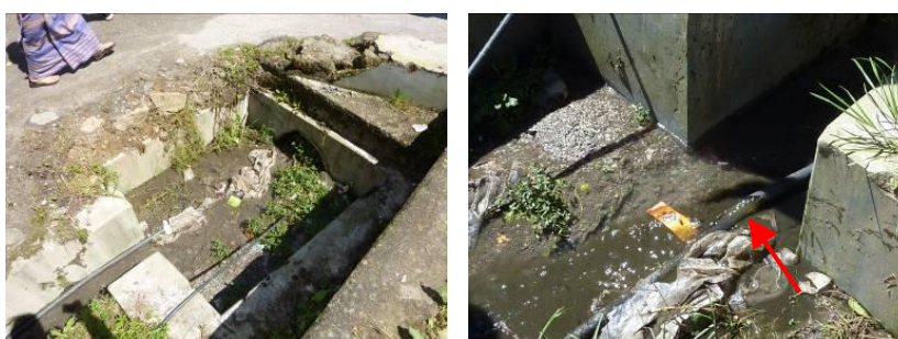
Figure 7: Discharge pipe of septic tank with accumulated sludge (unclogged by the assessment team)
