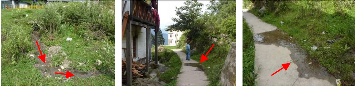
Figure 22: Improper drainage of grey water
