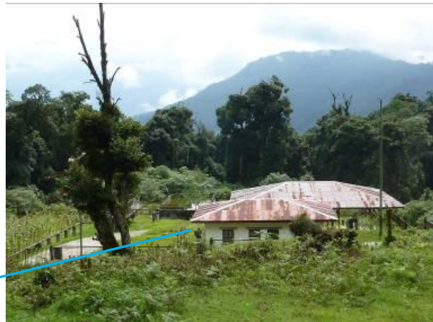
Figure 23: View of the sewage treatment plant
