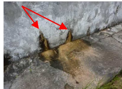
Figure 33: Cracks in the structure of one oxidation ditch
